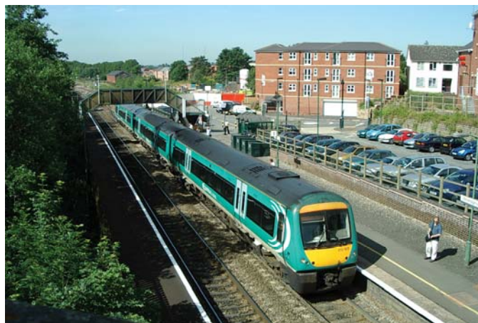
Figure 34: Bromsgrove Train Station
